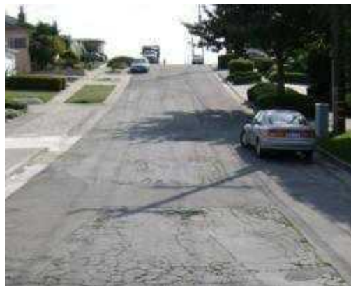
Figure 26: Inconsistent road surface 24
