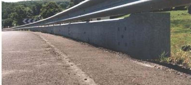
*On a French road, a second lower flat rail is fitted under the armco
