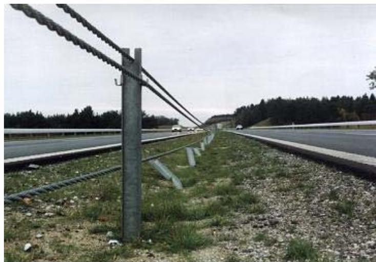
*Wire Rope Safety Fence: here, one of the cables is not in place, following an accident*
